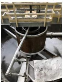
Figure 5: Primary Clarifier Mechanism
