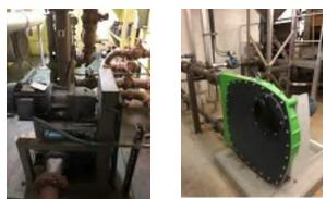
Figure 19 and Figure 20: Sludge Feed Pumps
