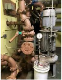
Figure 21: Sludge Transfer Pump
