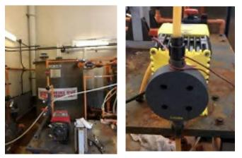
Figure 17: Ferric Chloride System
